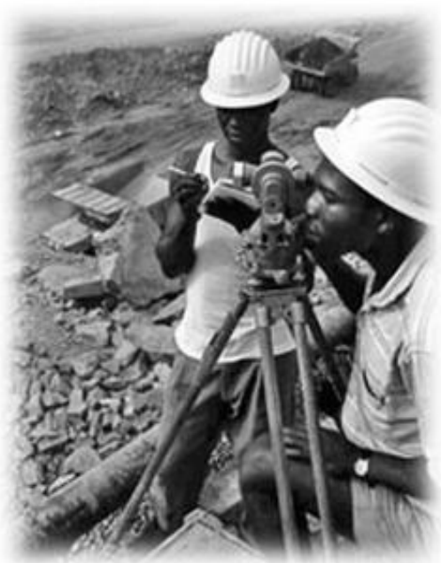
Two Ghanaian surveyors take a reading at the dam site, 1963
