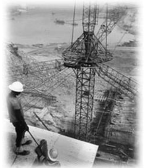
Construction work proceeds on the dam site, 1963
